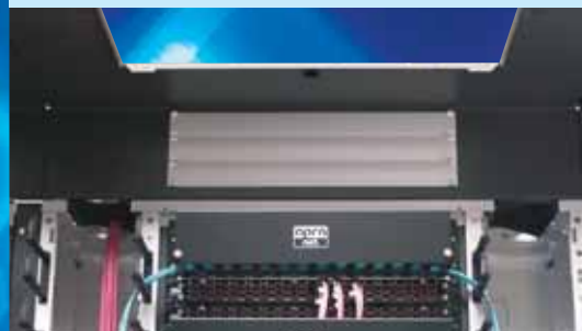
Internal view cooling corridor
